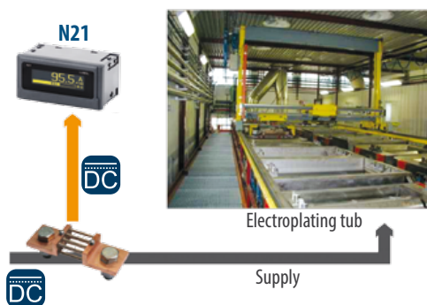
Current measurement in an electroplating plant
